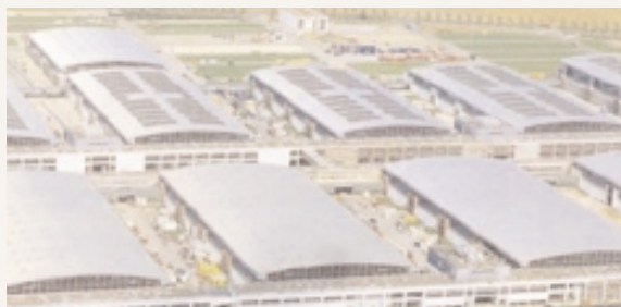
E.ON: Rooftop solar panel at the New Munich Trade Fair Center
