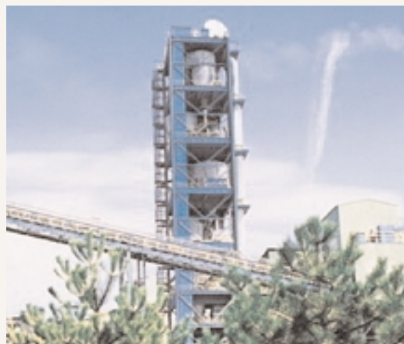
Lafarge: Cement plant at Cizkovice in the Czech Republic
