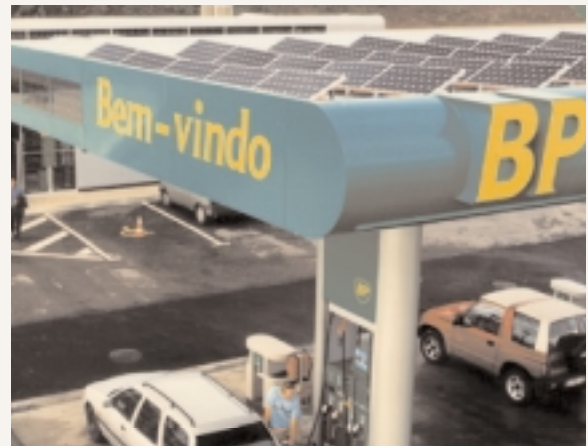
BP: Service Station in Portugal using solar panels for energy
